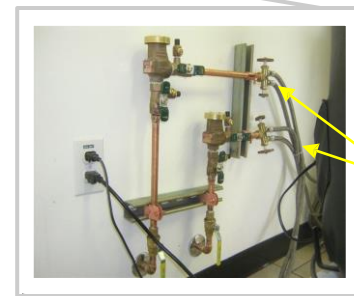
Typical PVB Installation
